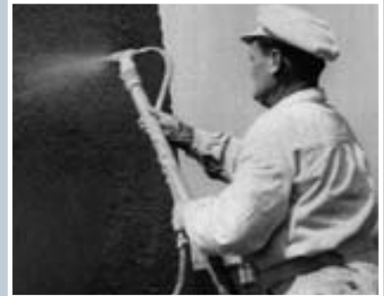
The first end hose spraying device still had a lot of rebound
