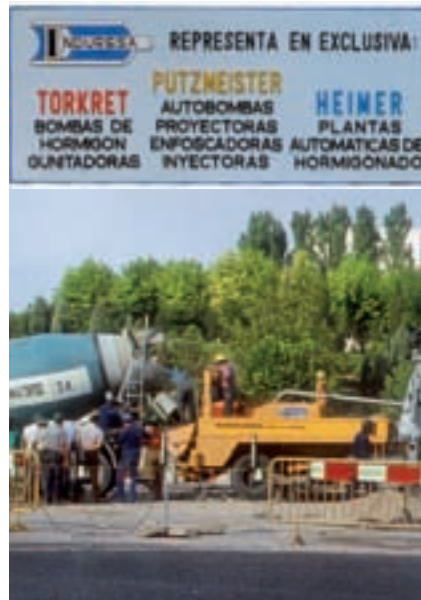
Putzmeister truck-mounted concrete pump B 232 S with "concrete crane" W 17/20 (Madrid 1971). Above, a plate with the names of the companies, which Induresa represented at the time. (Ill. Lettner)
