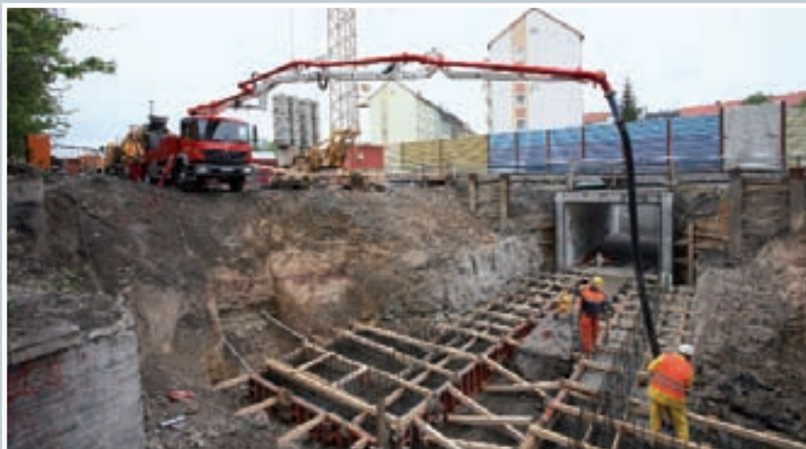
The M 20-4 introduced in 2005 is favoured on cramped construction sites with difficult access
