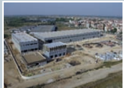
The newly constructed Putzmeister works in Turkey
