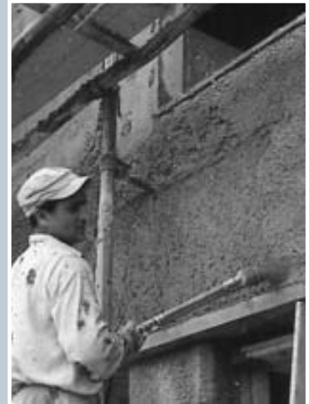
Plastering job with sharp, clean sprayed steel
