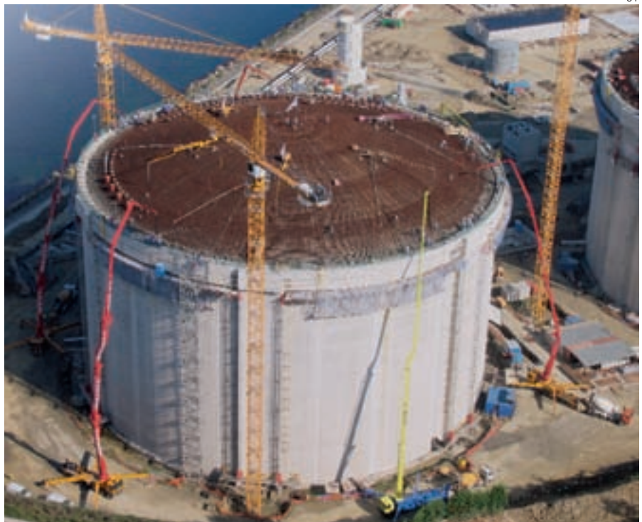
60-metre long-reach boom pumps during concreting of gigantic liquid gas tanks in Northern Spain
