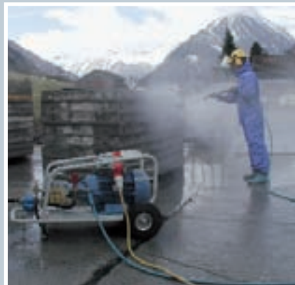
Formwork cleaning with Dynajet at 350 bar
