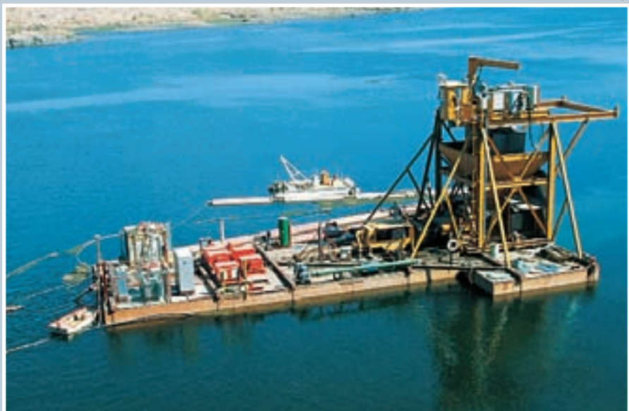
Use of a stationary concrete pump during sludge removal at the Aswan Dam
