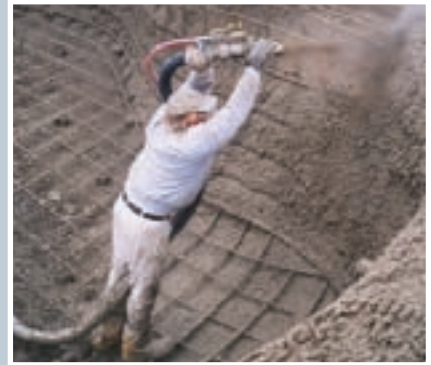
"Guniting" is widespread in the USA
