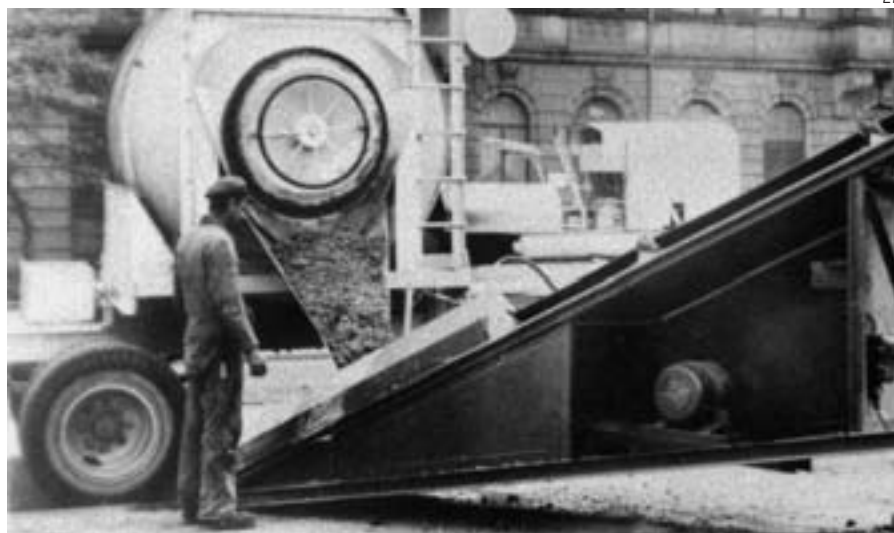
Transporting concrete by conveyor belt, 1934 (Ill. Verlag Bau+Technik)
