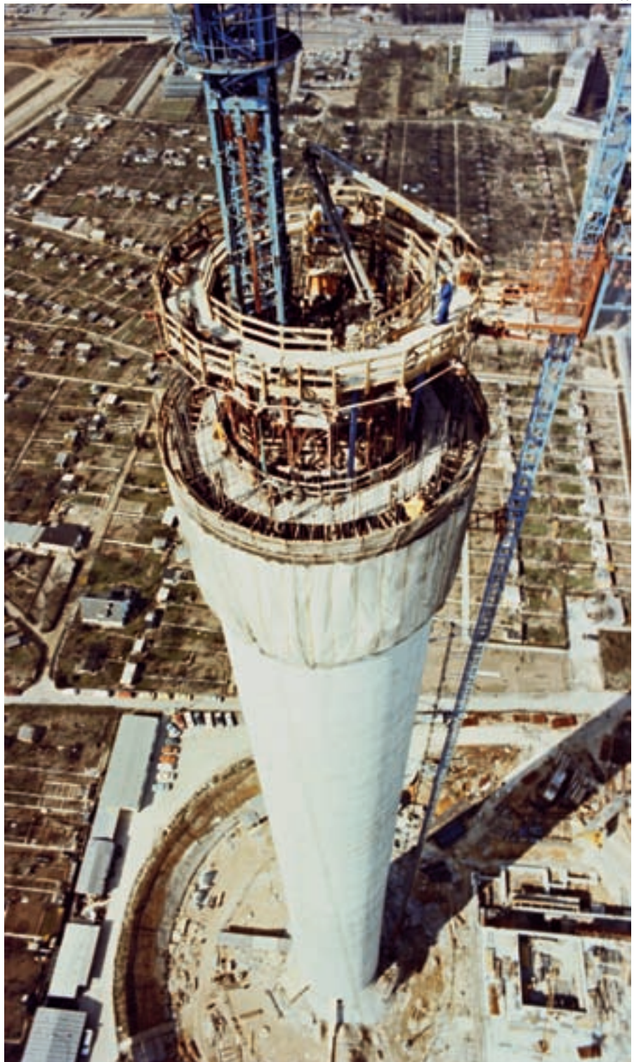
On the Frankfurt telecommunications tower, the concrete was actually supposed to be hoisted in the crane bucket. But something else happened ...
