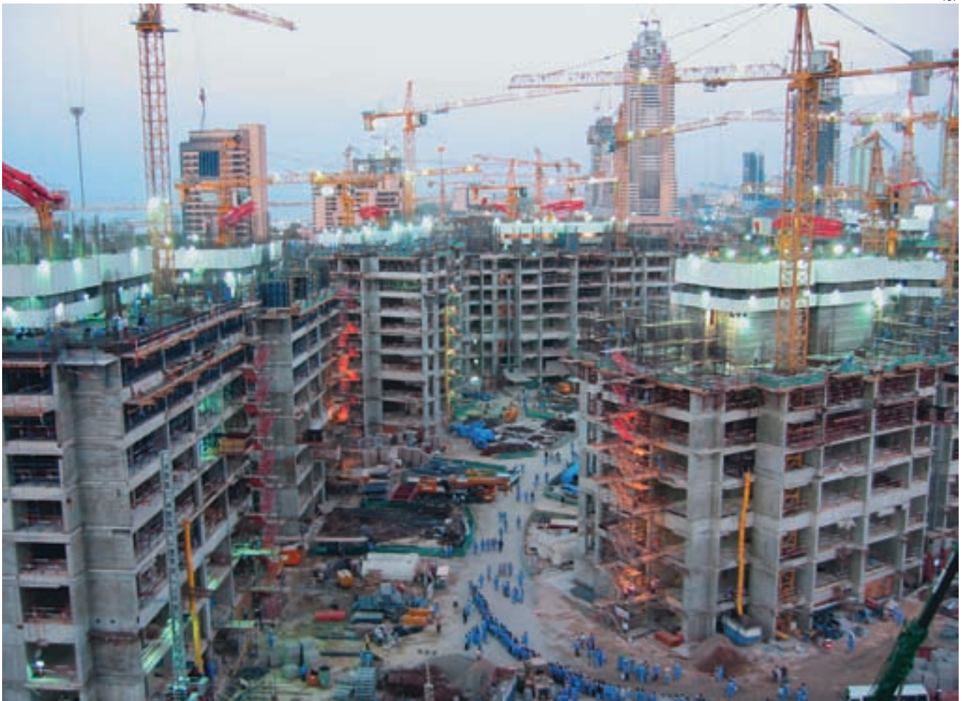
On the numerous high-rise construction sites in the Emirates, not only Putzmeister concrete pumps, but also stationary concrete placing booms are used
