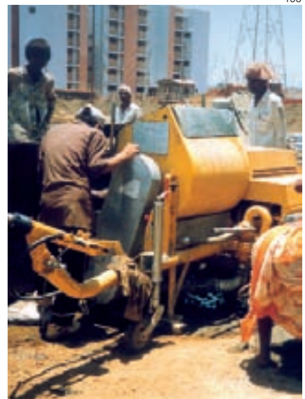
Putzmeister P 13 mortar pump on a construction site in the Gulf
