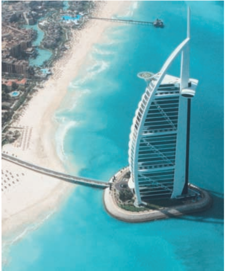
The façade of the 321 m high 7-star hotel Burj al Arab is based on the sail of a dhow (Arabic cargo boat). The concreting was performed using a stationary Putzmeister concrete pump, serviced by German Gulf
