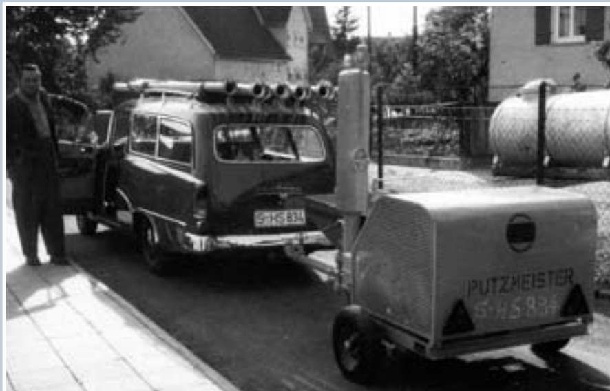
Mortar pump P1 with sprinkling pipes for mortar delivery (“mortar conductor”)
