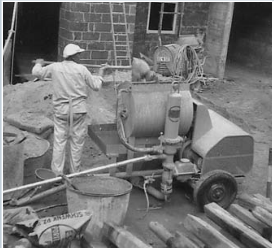
The successful Putzmeister model PKM with integrated pugmill mixer and diesel engine
