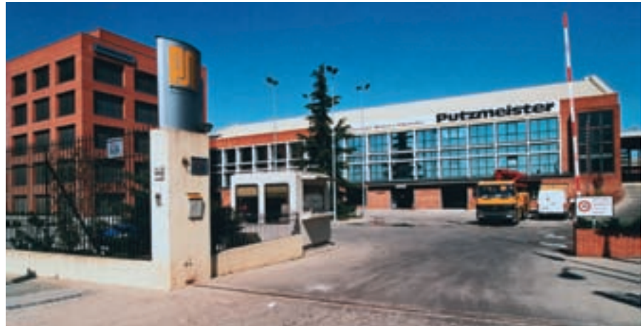
Management, after-sales service and assembly at Putzmeister Ibérica have since been housed in new or renovated buildings (2004)
