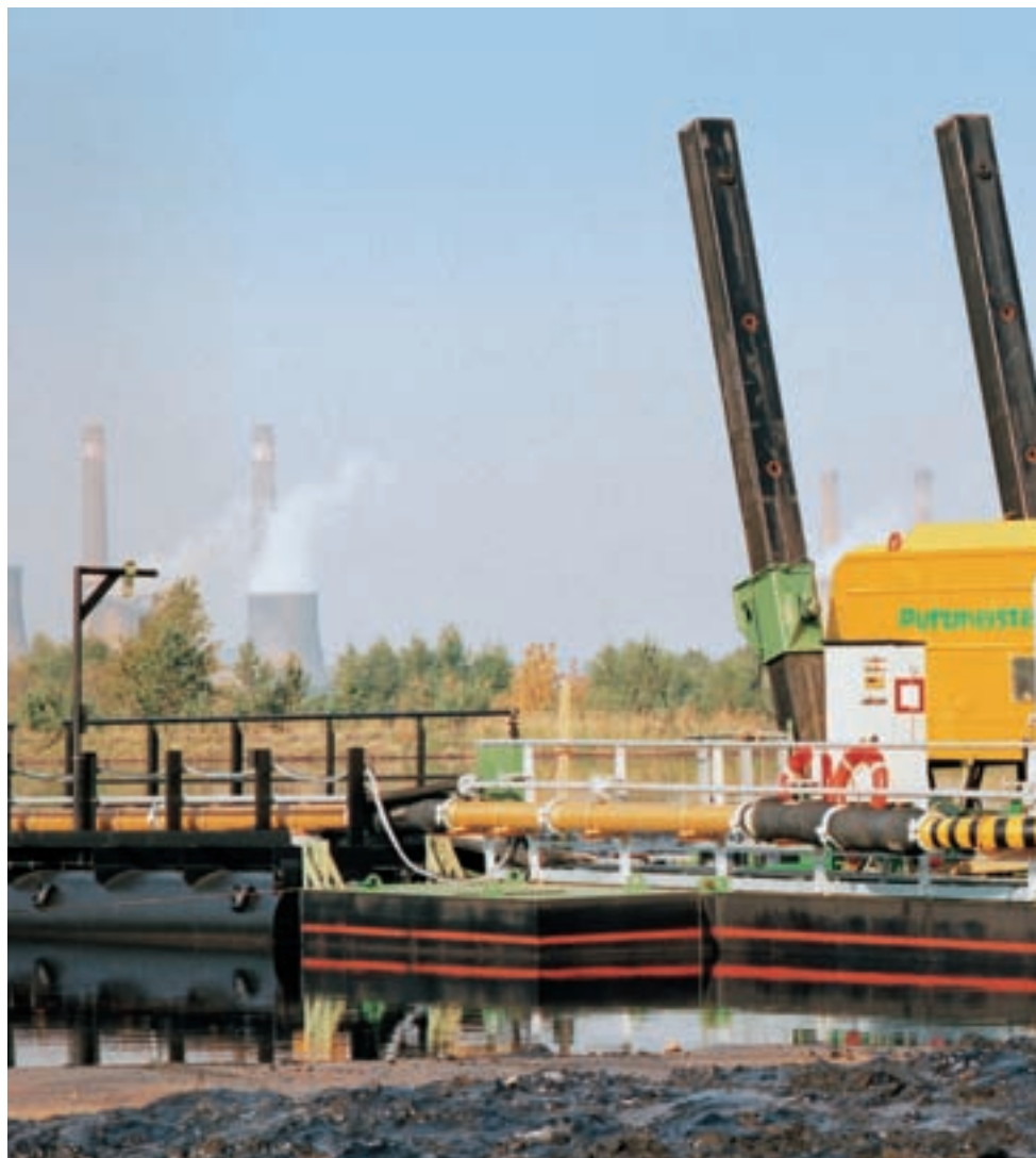
The 500,000 tons of toxic, sticky creosote solid mixture containing phenol from a former repository were pumped using Putzmeister pumping technology into a treatment plant
