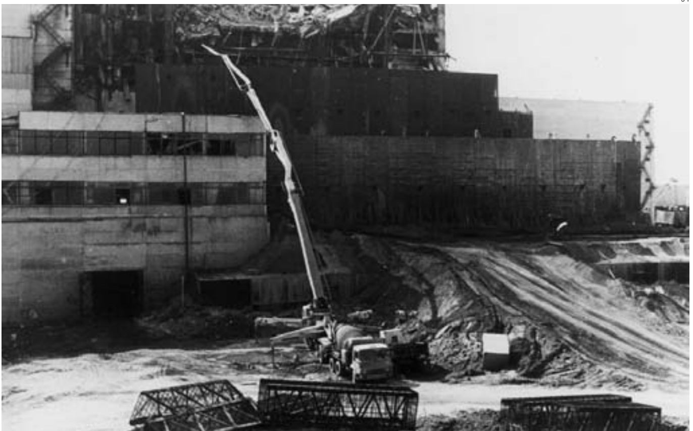
The Putzmeister large boom pumps were either fed from several hundred metres away by stationary concrete pumps or – as here – directly from truck mixers
