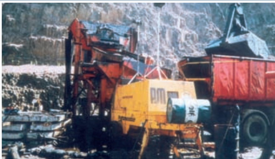
Oil sludge, sand, stones and flotsam were pumped by these concrete pumps, before the mud reached a seawater desalination plant
