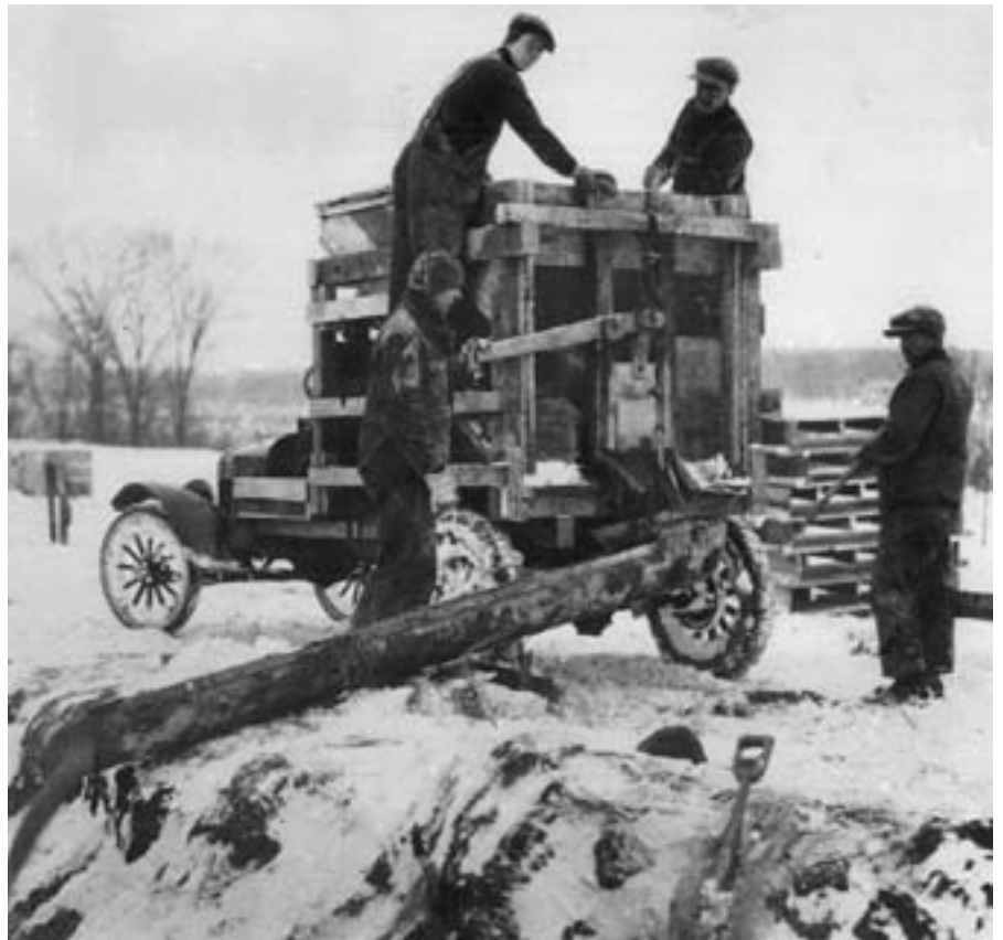
Truck-mounted concrete transporter as forerunners of the concrete mixer, USA 1924 (Ill. Ford Motor Co.)
