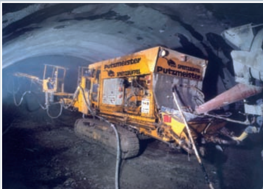
Twin shotcrete buffalo on a tunnel construction site for a new high speed line of German railway
