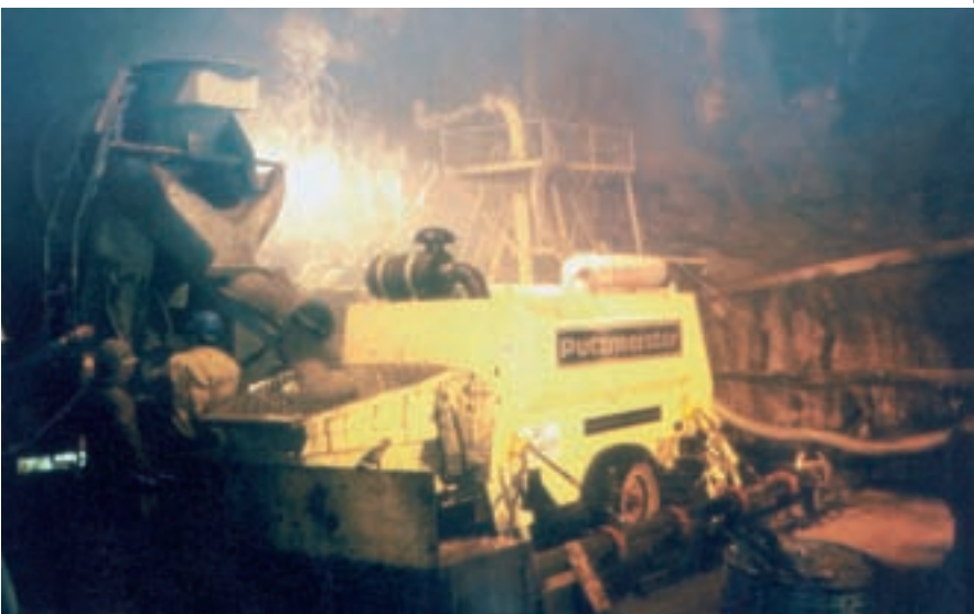
In February 1985, this stationary concrete pump with S transfer tube (see also page 26) improved on the world record for high-rise concrete pumping to 432 m in the Spanish Pyrenees
