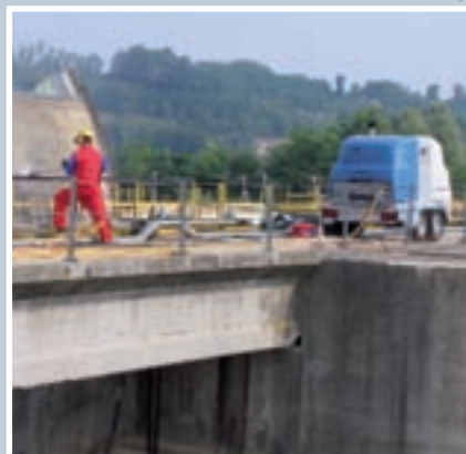
Dynajet high-pressure cleaner UHP 170 during coating removal at 2,800 bar
