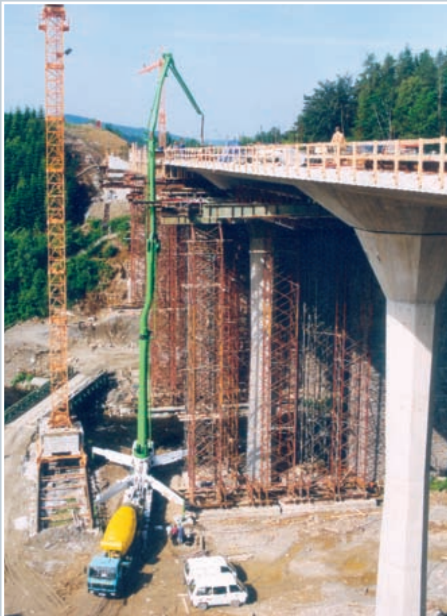
Concrete placing booms with five sections offer a considerably more flexible working range. Above a Putzmeister M 52-5, below a M 62-5 (first generation, 1986).
