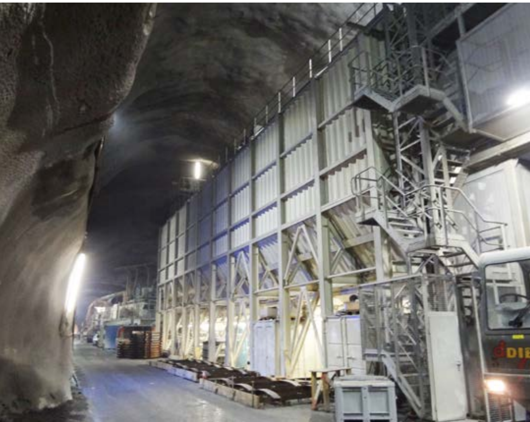
▲ The concrete batch plant is underground. The stationary concrete pump is placed under the mixer and pumps the concrete 450 m into the machine cavern.
