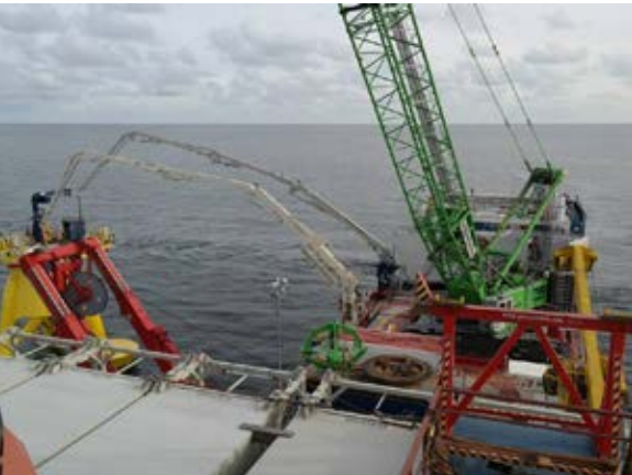
▲ Two MX 32-4 concreting a foundation from the ship
