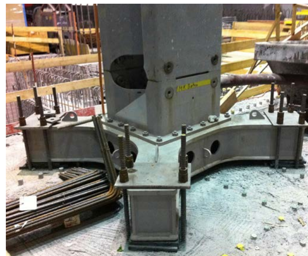
▼ The MX 32-4 in the machine hall sits on the X base and is fixed to the base plate with tie rods.
