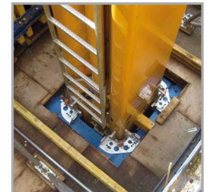
Tubular column with slab guide
