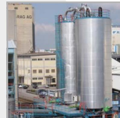
Two 200 m<sup>3</sup> storage silos for sewage sludge storage (Pro Rheno, Switzerland)
