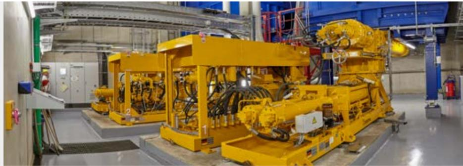
Two sewage sludge reception bunkers of 60 m<sup>3</sup> each with sliding-frame extraction system, double-shaft bunker discharge screw conveyors, KOS 1080 HP high-density solids pump
