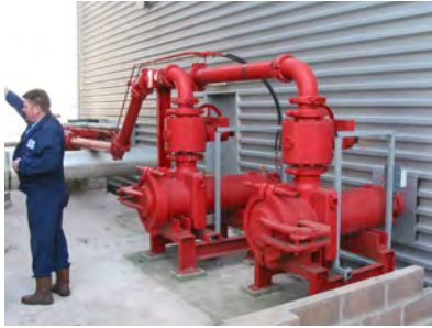
Fig. right 124: Foreign body separator with demountable trolley; the trolley makes the extraction of the basket easier
