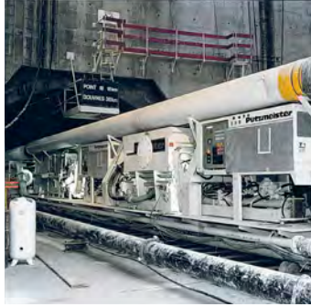
Fig. 64: One of eight muck pumps during the construction of the Euro Tunnel between France and England
