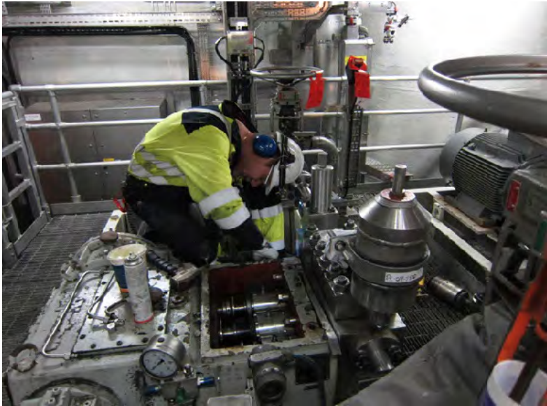
Fig. 75: Plunger pump
