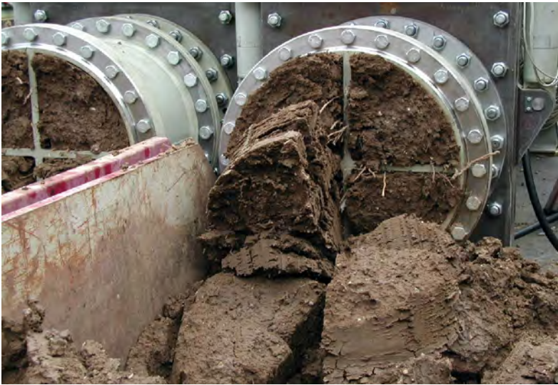
Fig. 67: Excavated muck; the material plug is easy to recognize
