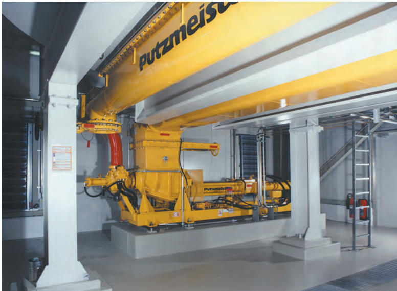
Fig. 120: Silo discharge screw feed the solid pump
