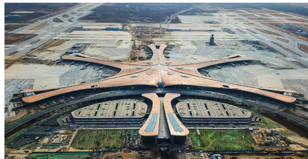
Beijing Daxing International Airport, China
