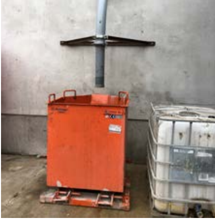
Cleaning line for concrete residue and cleaning water outside the hall
