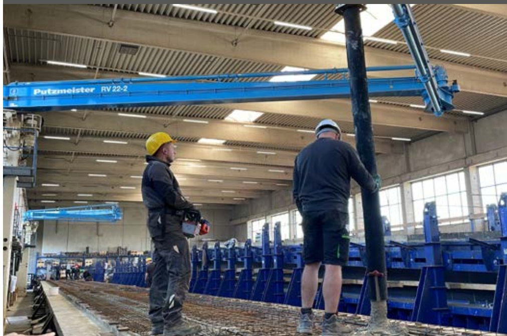
Concreting of Pi ceilings with rotary distributor RV 22-2
