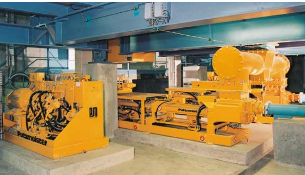
Two high density solids pumps KOS 1030 with HA 22 for charging sewage sludge into the refuse incinerator at Dinan, France
