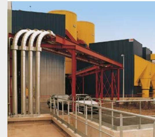
Insulated delivery lines from the reception to the incinerator building
