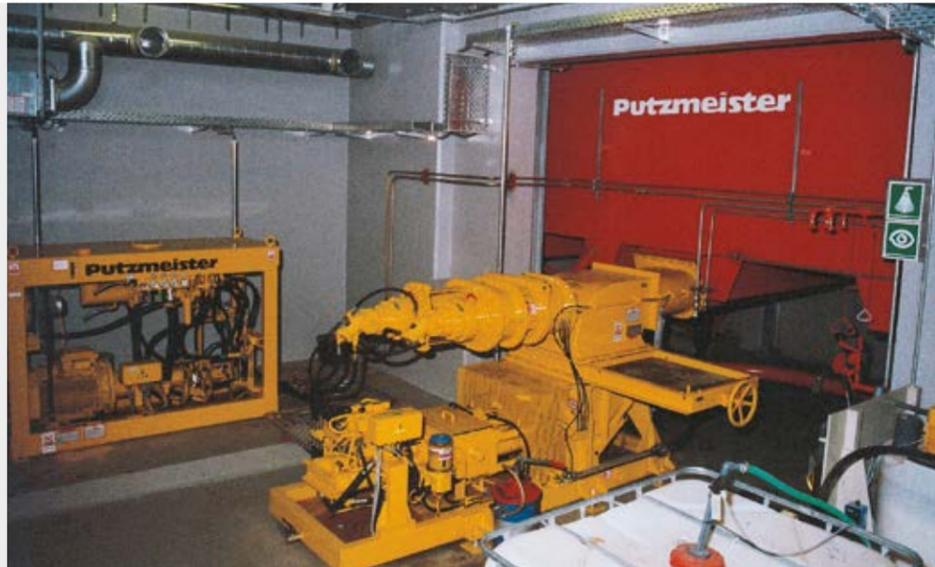
**Above:** 60 m<sup>3</sup> reception silo with injection pump KOS 540 and power pack HA 45 in the refuse heating and power station at Vestkraft, Copenhagen, Denmark
