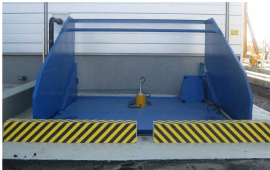
Receiving bunker to receive sludge by trucks from an intermediate emergency storage
