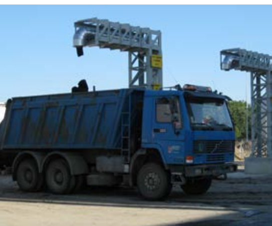
Emergency truck loading station
