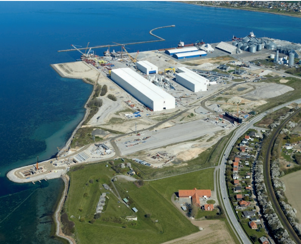
Fig. 2: The three production halls for manufacturing the precast elements for the Storstøm Bridge. (copyright: Vejdirektoratet)
