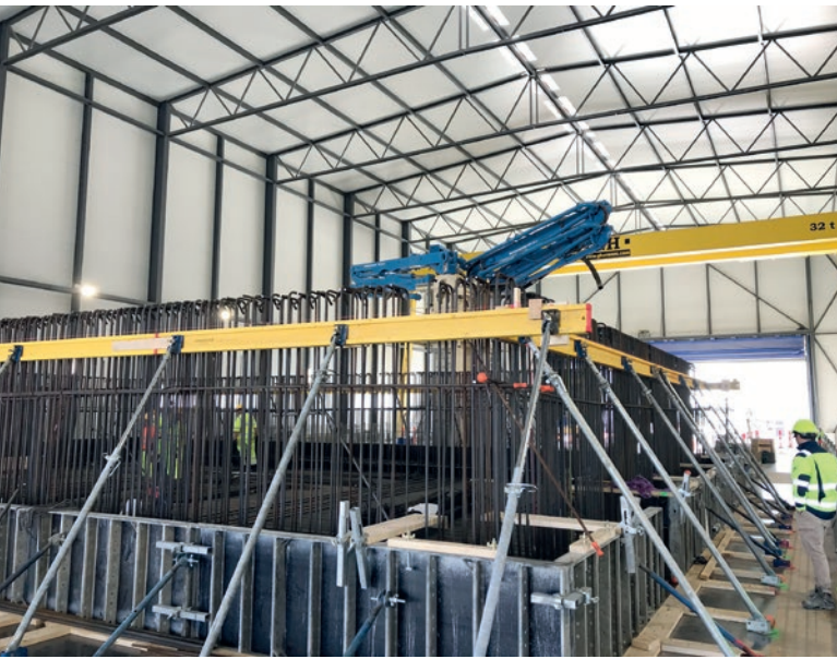
Fig. 5 and 6: Reinforcement cage of the first foundation element (left) and the two MX24 distribution masts on the tubular column system (right).
