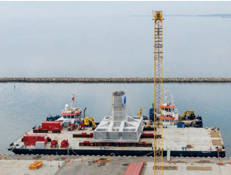
Fig. 7: Completed foundation, ready for transport (copyright: Vejdirektoratet)
