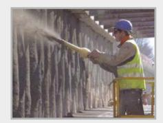
Fine concrete pumps like the P 715 are among the most versatile systems. You can use them for shotcrete or for pumping fine concrete with a grain size of up to 16 mm.
