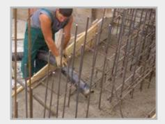
Fine concrete pumps like the P 718 are among the most versatile systems. You can use them for shotcrete or for pumping fine concrete of up to 32 mm.
