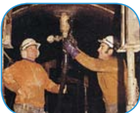
Grout injection and backfilling
