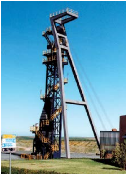
Winding tower of the Hajar mine
