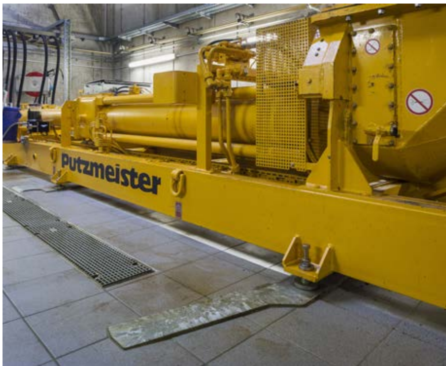
Innovation for maintenance: The KOS is simply swivelled out on plates installed on the ground
