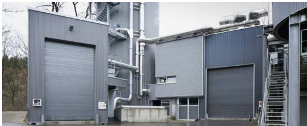
Every year up to 60,000 t of external dewatered sewage sludge is hauled from the surrounding communities
