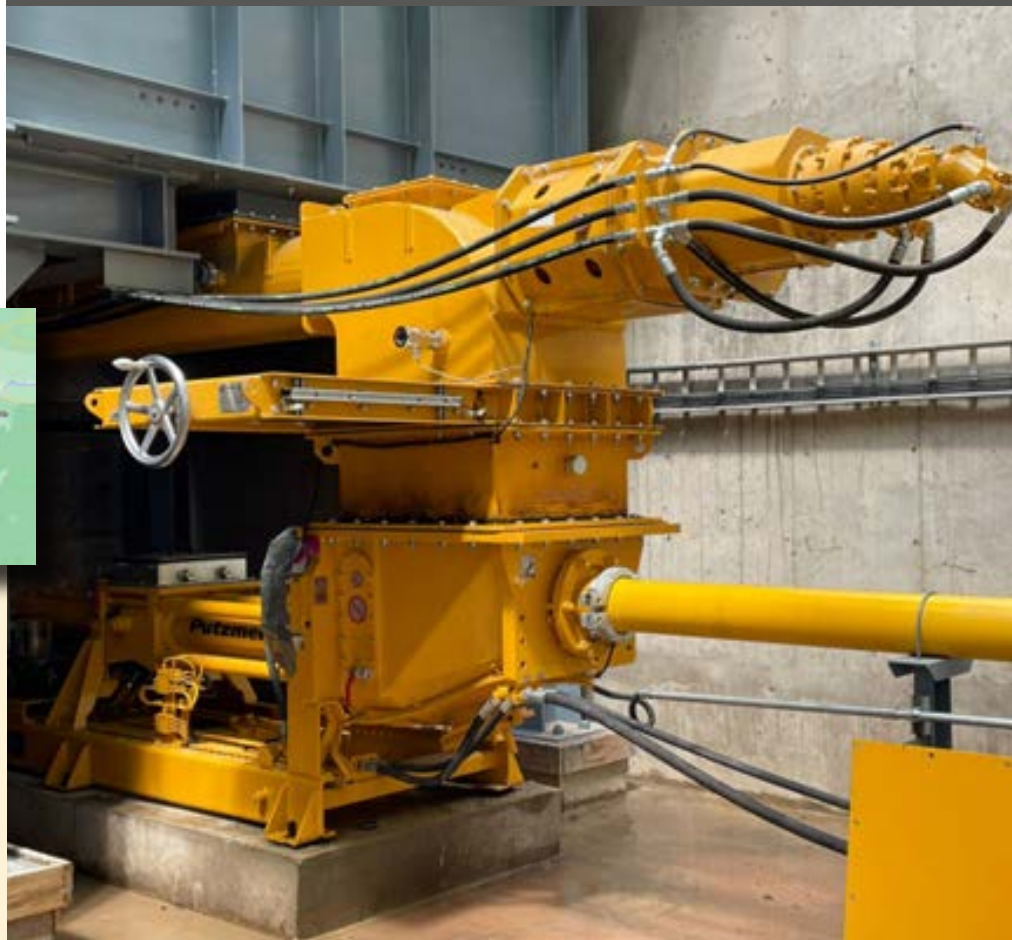
KOS high density solids pump with S-tube technology under crane drop bunker
