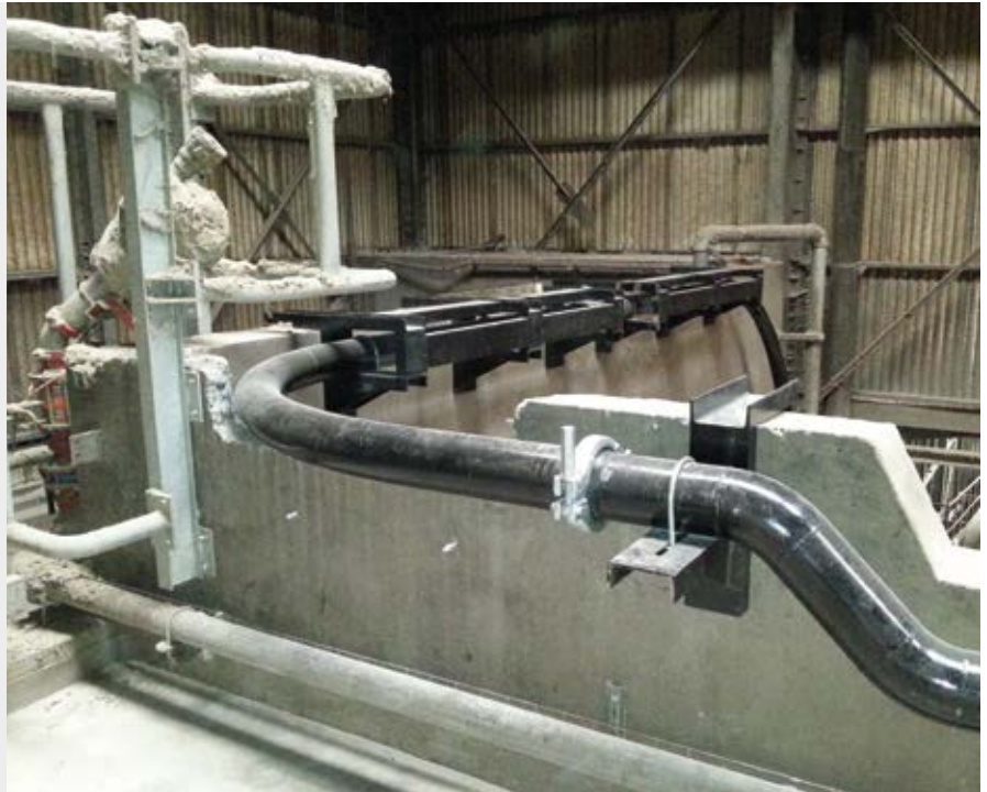
Sludge delivery line with Putzmeister ZX coupling system
