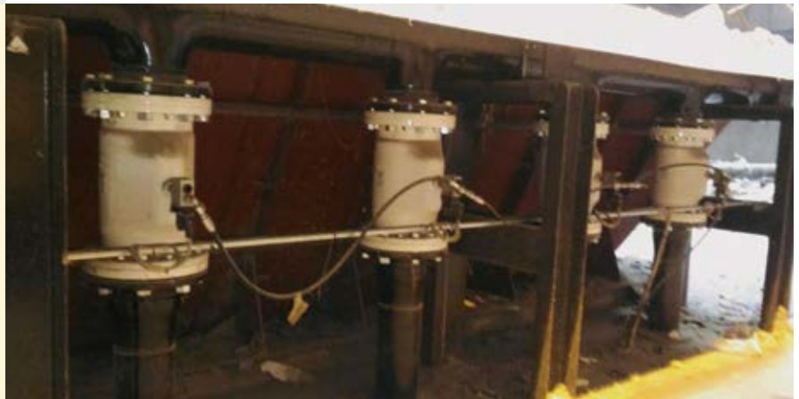
The sludge is distributed by 4 pinch valves to the hopper of the kiln
