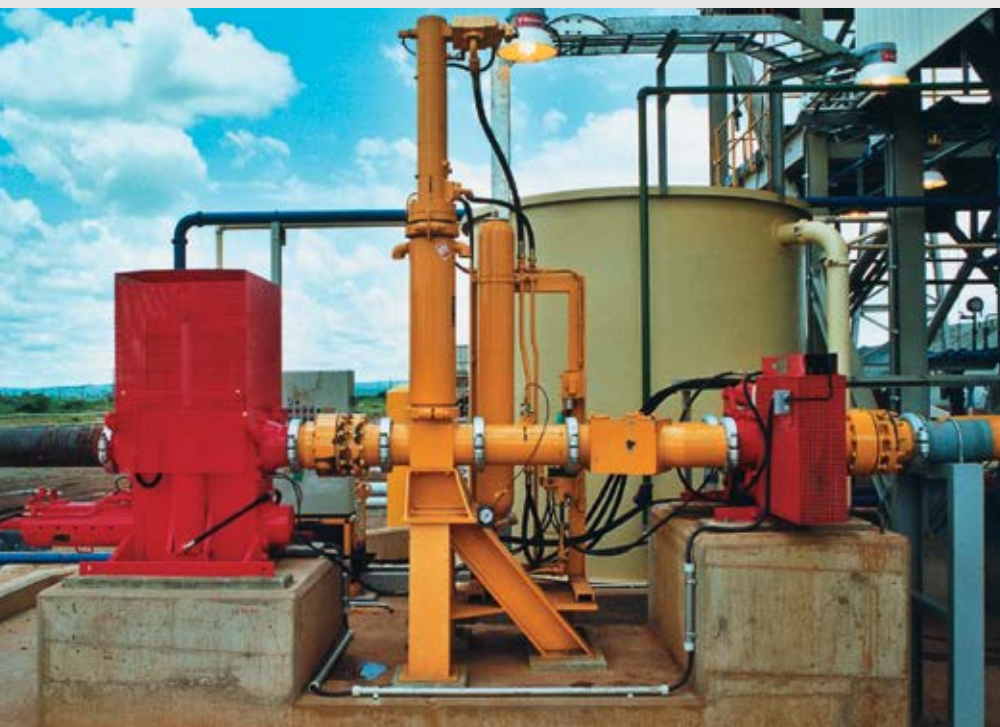
The pig in gate ZX 200, the high pressure damper HPD 200/750 and the diversion valve DVH 4/2
