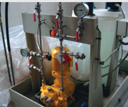
Above: BLI dosing station with mixing tank and control equipment
