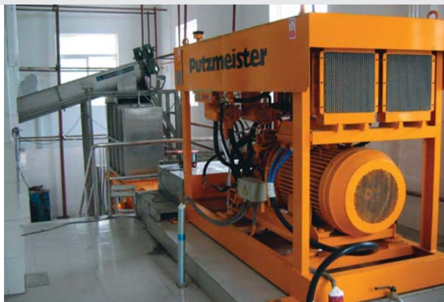
Above: BLI dosing station with mixing tank and control equipment
