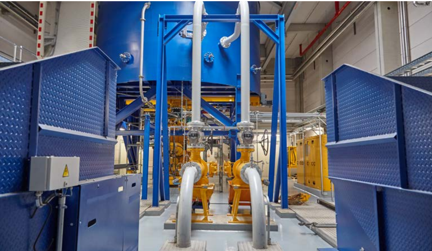
Foreign body separation upstream of the feed into the 1000 m 3 storage silo
