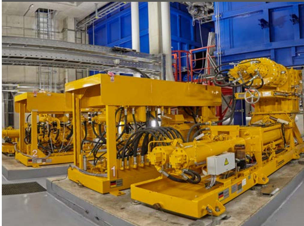
Two sewage sludge reception bunkers of 60 m 3 each with sliding-frame extraction system, double-shaft bunker discharge screw conveyors, KOS 1080 HP high-density solids pump
