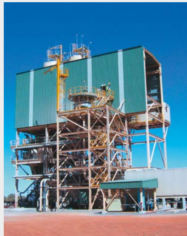
General view of paste treatment plant
