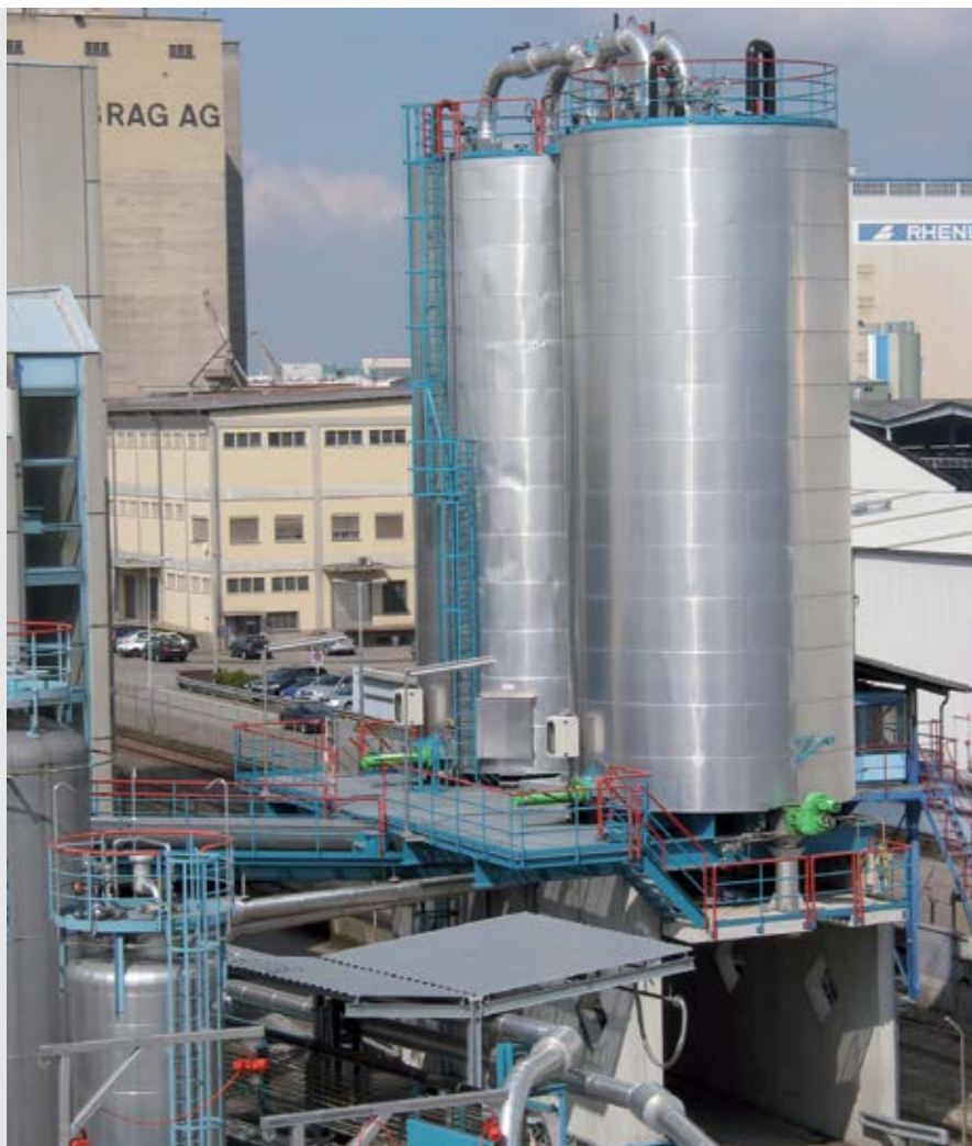
Above: Two storage silos (insulated), each holding 200 m 3 – for storing the sewage sludge
