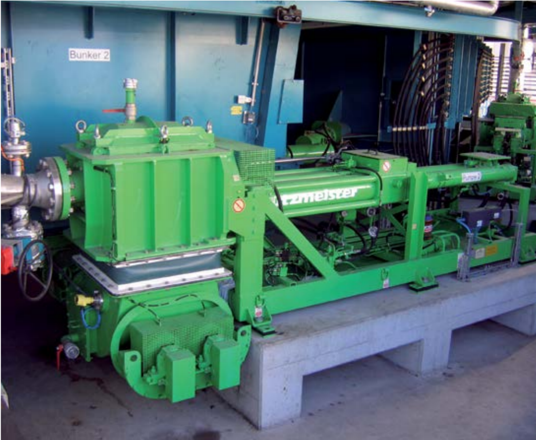
KOS 1470 high density solids pump in LCB version
