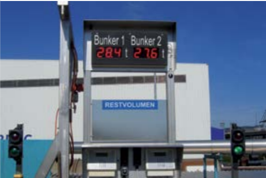
Above: Sludge reception bins 1 and 2 Below: Display of the quantity of sludge still present in the reception bin
