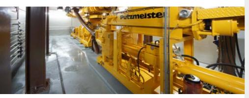
Background: KOS 1080 piston pump under a 30 m<sup>3</sup> receiving bunker. Foreground: KOS 1030 piston pump to feed the kiln lines under a 230 m<sup>3</sup> storage silo. Installed in a very narrow former waste bunker.
