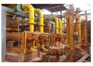
VPD system installed after a HSP piston pump for tailings handling
