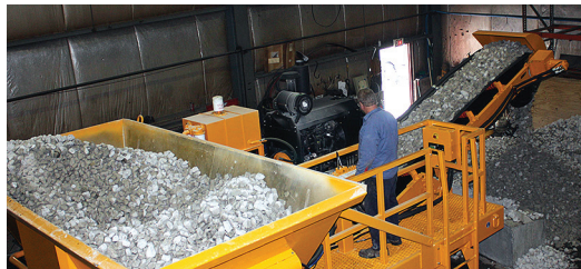
15 yd 3 (12m 3 ) capacity hopper loaded with 3" (76.20mm) diameter aggregate. Hopper can discharge material at rates up to 6 yd 3 /min (4.8m 3 /min). Operator is conveniently located to safely observe charging of hopper, feeding onto belt, and rate of discharge.
